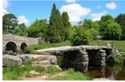
The Old Clapper Bridge, Postbridge
