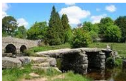
The Old Clapper Bridge, Postbridge
